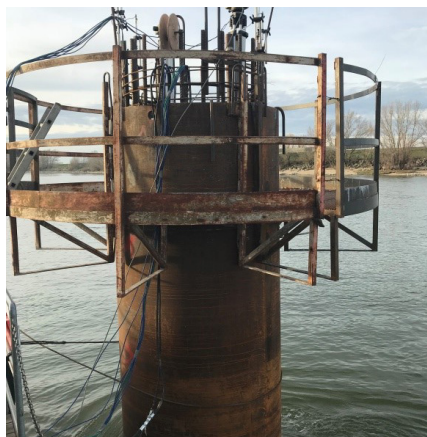
Pile under test.
