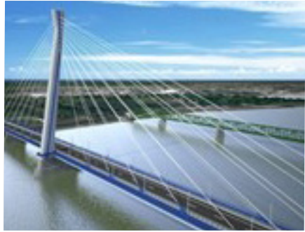
The 600m bridge will improve road connectivity between Hungary and Slovakia (photo: Pont-Terv engineering consultants).
