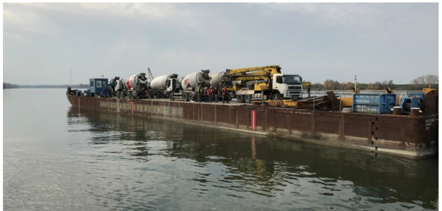
Concrete was delivered to the mid-river site by barge.
