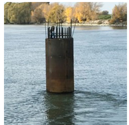
Pile after installation.
